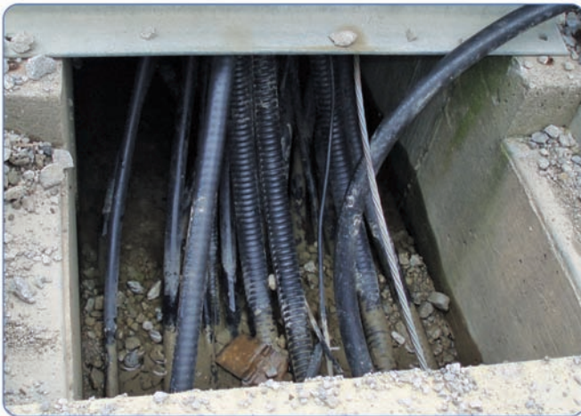
Figure 2. Traditional cable trenches
